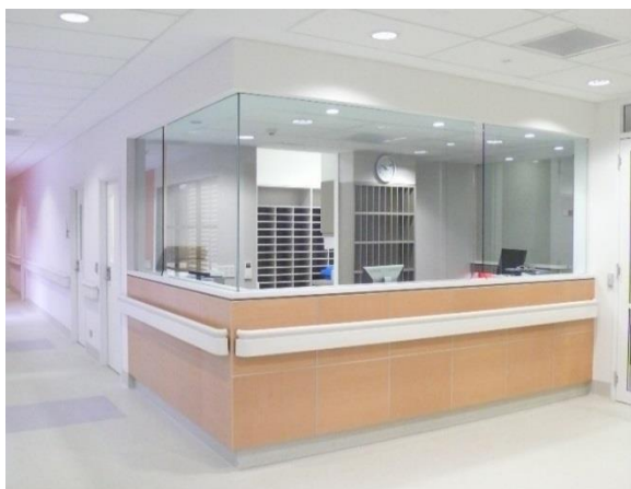
Figure 4.5: Staff Station with security glazing barrier
