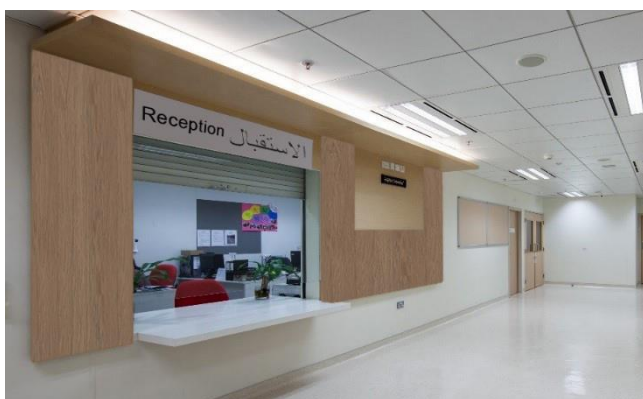
Figure 4.7: Reception with vertical roller shutter for after-hours security
